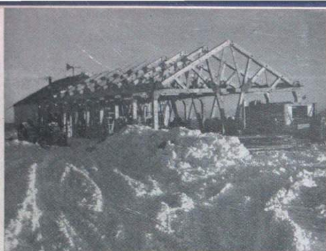
Most of the trusses and framework up, with the one end finished where we were living
