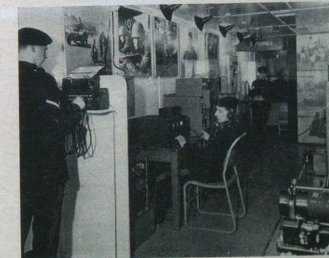
Part of the interior of "Quicksilver." Lance-Corporal Davies at the switchboard, Lance-Corporal Bowden operating the WS 53 and Sergeant Topan at the Enquiring desk
