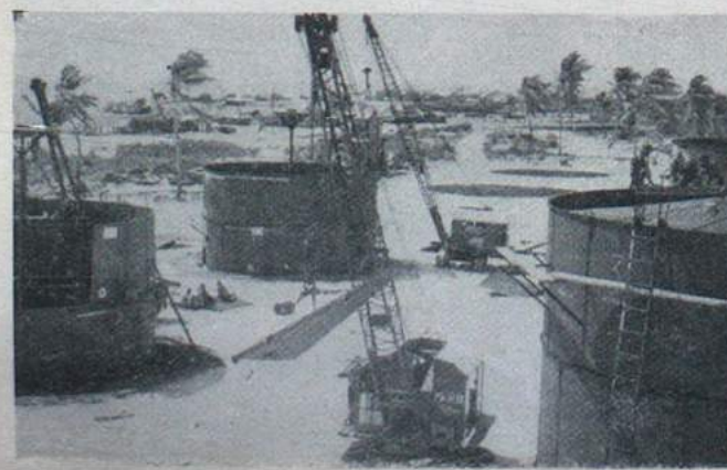
● Construction of the Tank Farm at "Port London"
