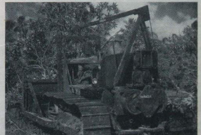
Bulldozer clearing the cable route
