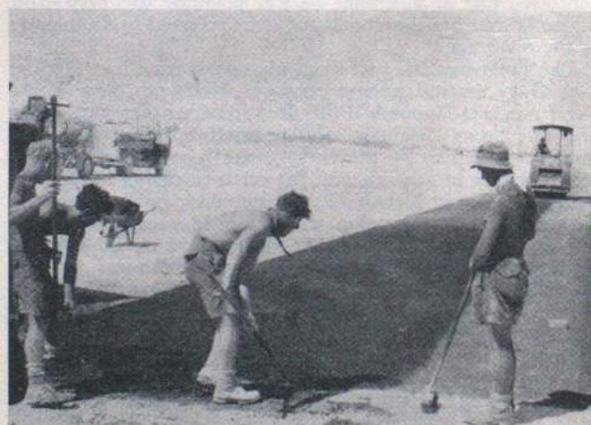
● Laying the first strips of asphalt on the runway
