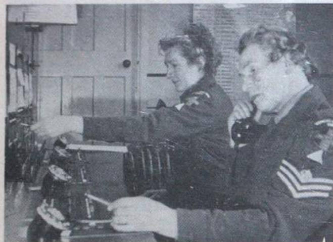
Switchboard Operating. Staff Sergeant Neale and Private Lester (W.R.A.C.). No. 2 Northern Comd. (M) Sig. Regt. (T.A.)
