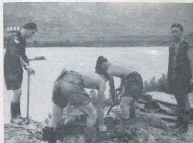
KAM TIN BRIDGE
